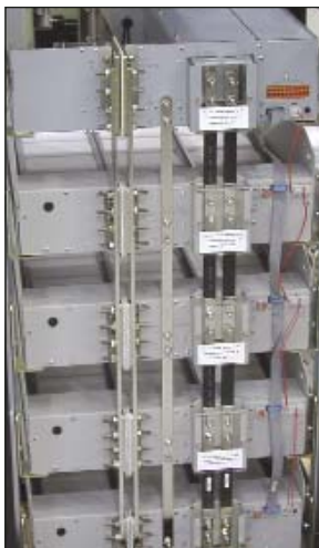
Integrated System Bussing & Alarm Connections
